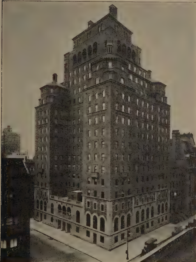
719 Murgatroyd and Ogden, architects; photograph by Wurts Brothers
